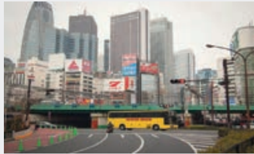
01 - Day view, the bridge before Kabukichō District
